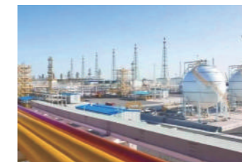
Petroleum Gas Detection
