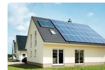
屋顶光伏系统 Rooftop photovoltaic systems
