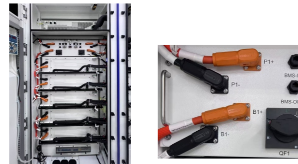
工商储Pack应用- 单芯大电流 Pack Application - ESS High Protection Connector
